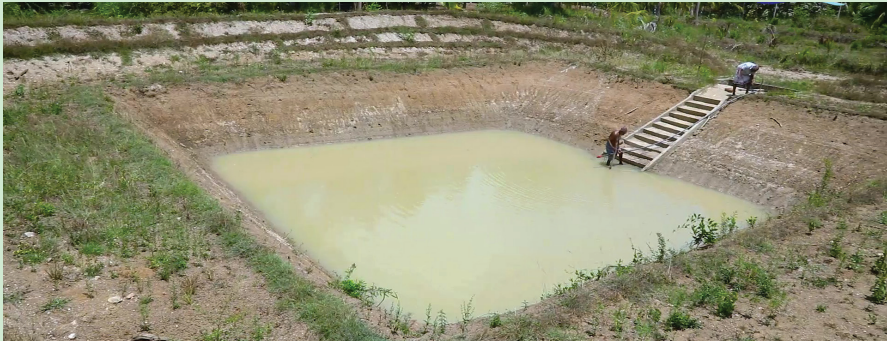
Runoff tank (Pathas) – Anguruwella Cascade, Kurunegala
