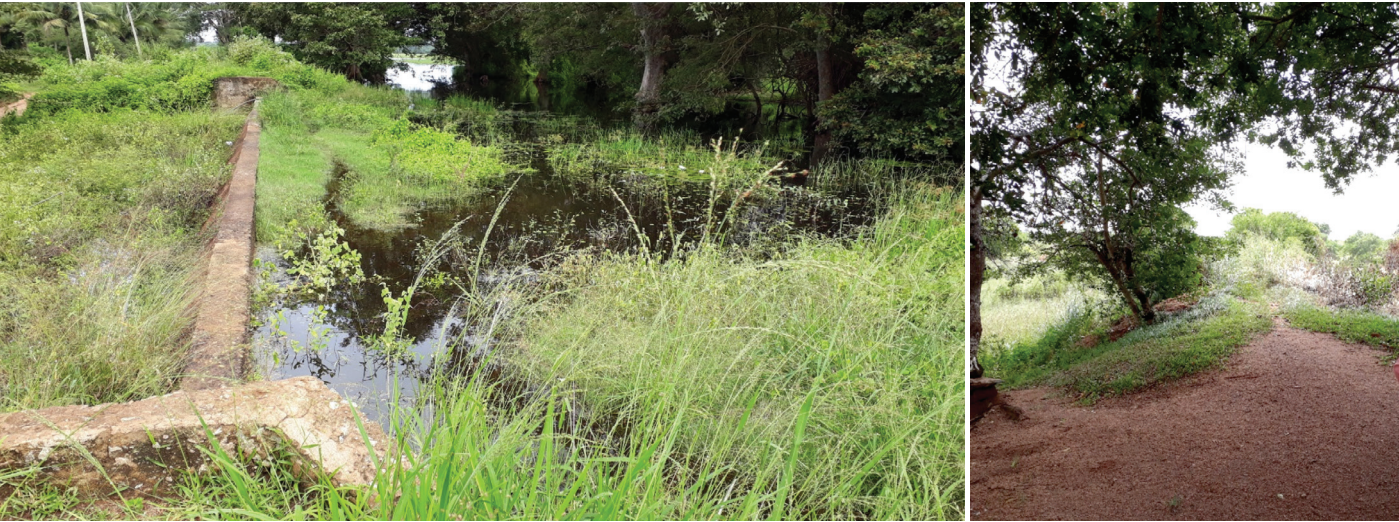
Figure 10: Poor maintenance of VISs: a major constraint to their sustainability
