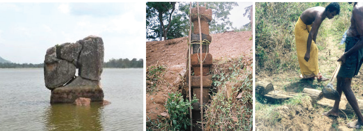
Figure 2: Remnants of ancient irrigation management structures a. Water depth measurement b. An ancient sluice structure c. Water flow measurement
