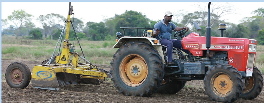
Laser leveling – Pahala Aliyawetuna Tank, Siwalakulama Cascade, Anuradhapura
